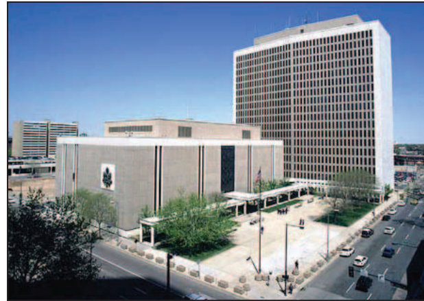
Photo provided by Bennett Wagner & Grody Architects
