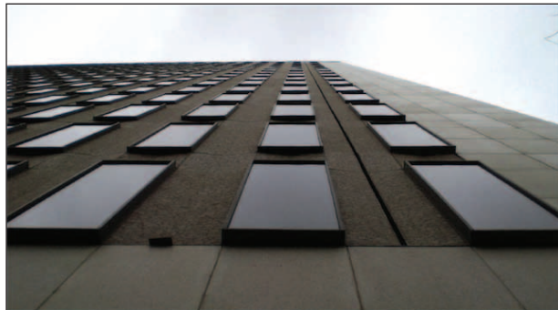
Photo provided by Bennett Wagner & Grody Architects
